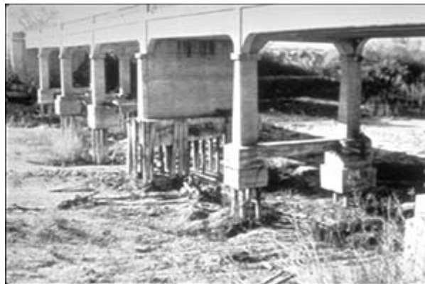
Figure 5-33 Effects of Bridge Scour
